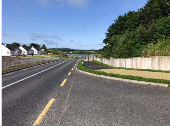
Figure 9 – N56 Looking south from the N56/L-6433
