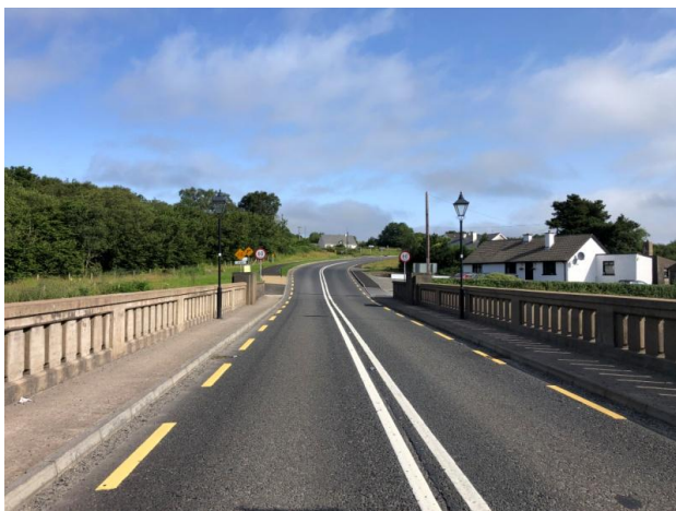
Fig 6 – N56 Gweebarra Bridge looking North
